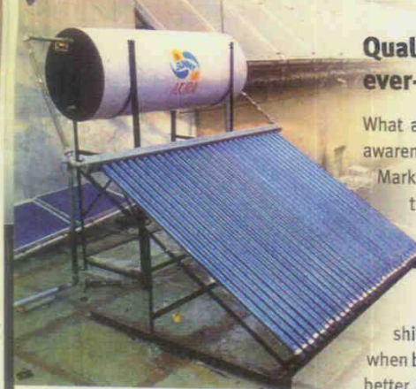
Thermosiphon system by NRG Technologists
